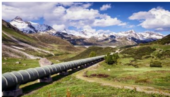
Supervision pipeline - failure, damage,...
