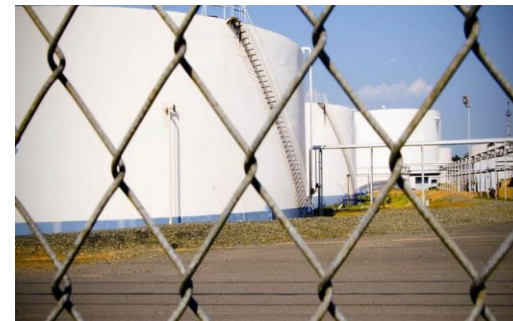
Localization of protective fencing
